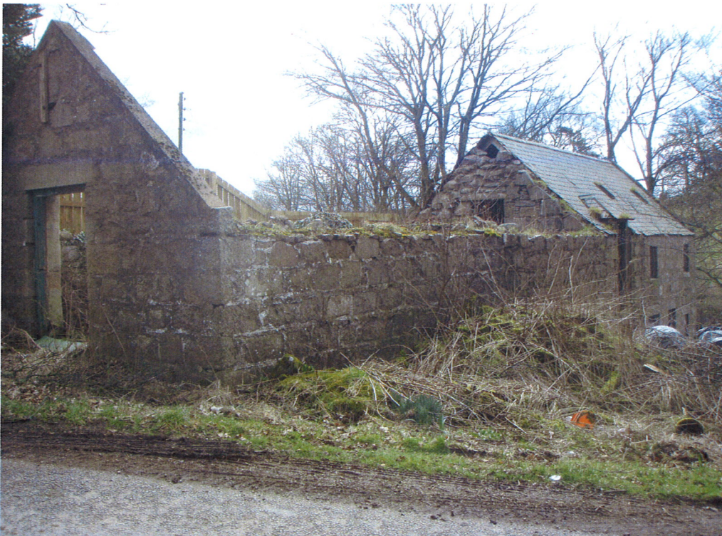
Photograph 2 – North West Elevation
