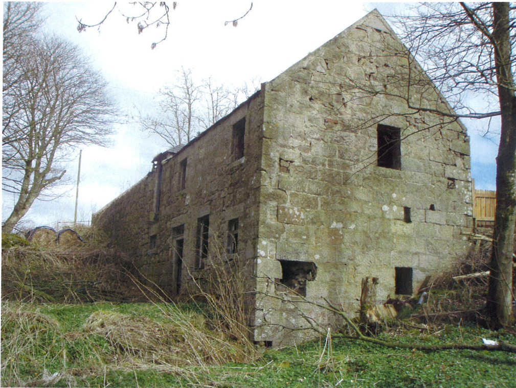
Photograph 3 – South West and North West Elevations
